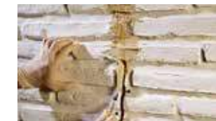
7- Covering the spaces by assembly putty by using a putty knife
