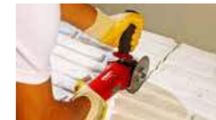
3- Cutting the panel by angle-grander
