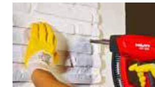
4-a) Assembling by nails
