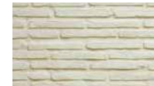
11- Installation finished after drying
