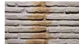
9- Waiting for drying for assembly putty
